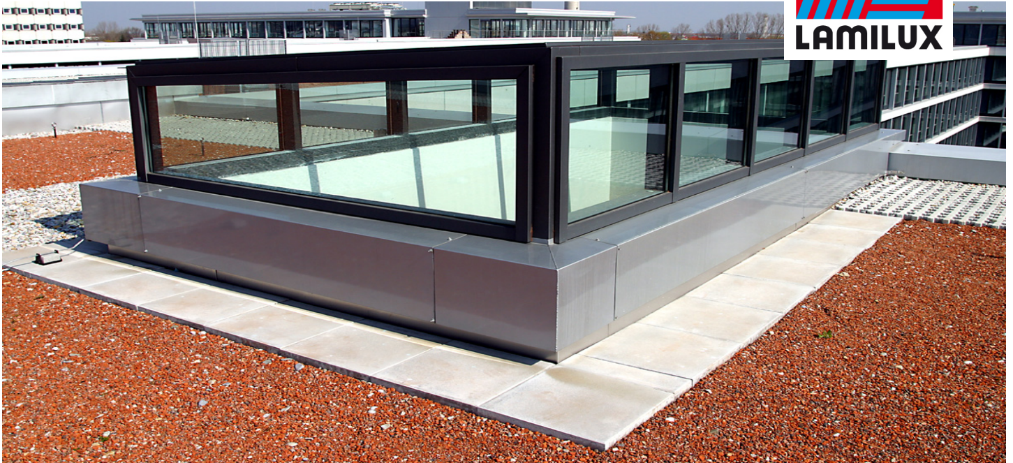
Parking facility, Schwabing
