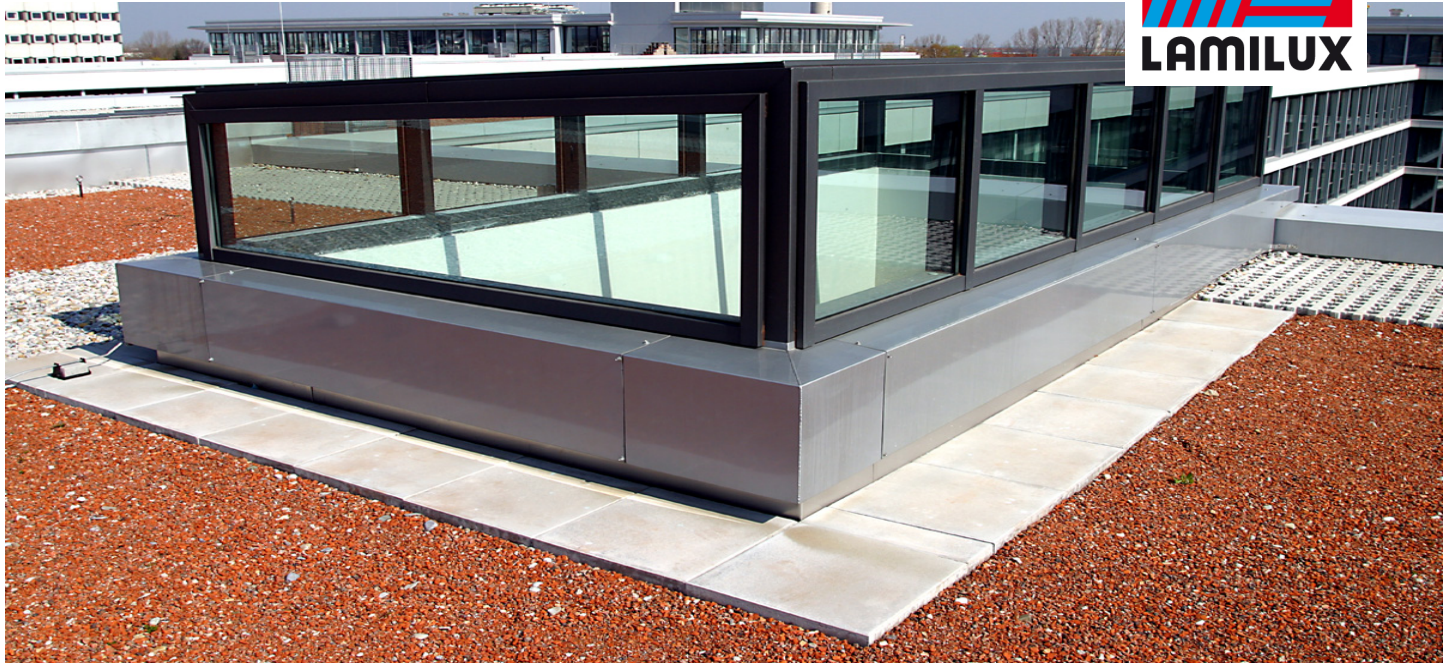
Parking facility, Schwabing
