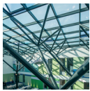
MIROTEC STEEL CONSTRUCTIONS
