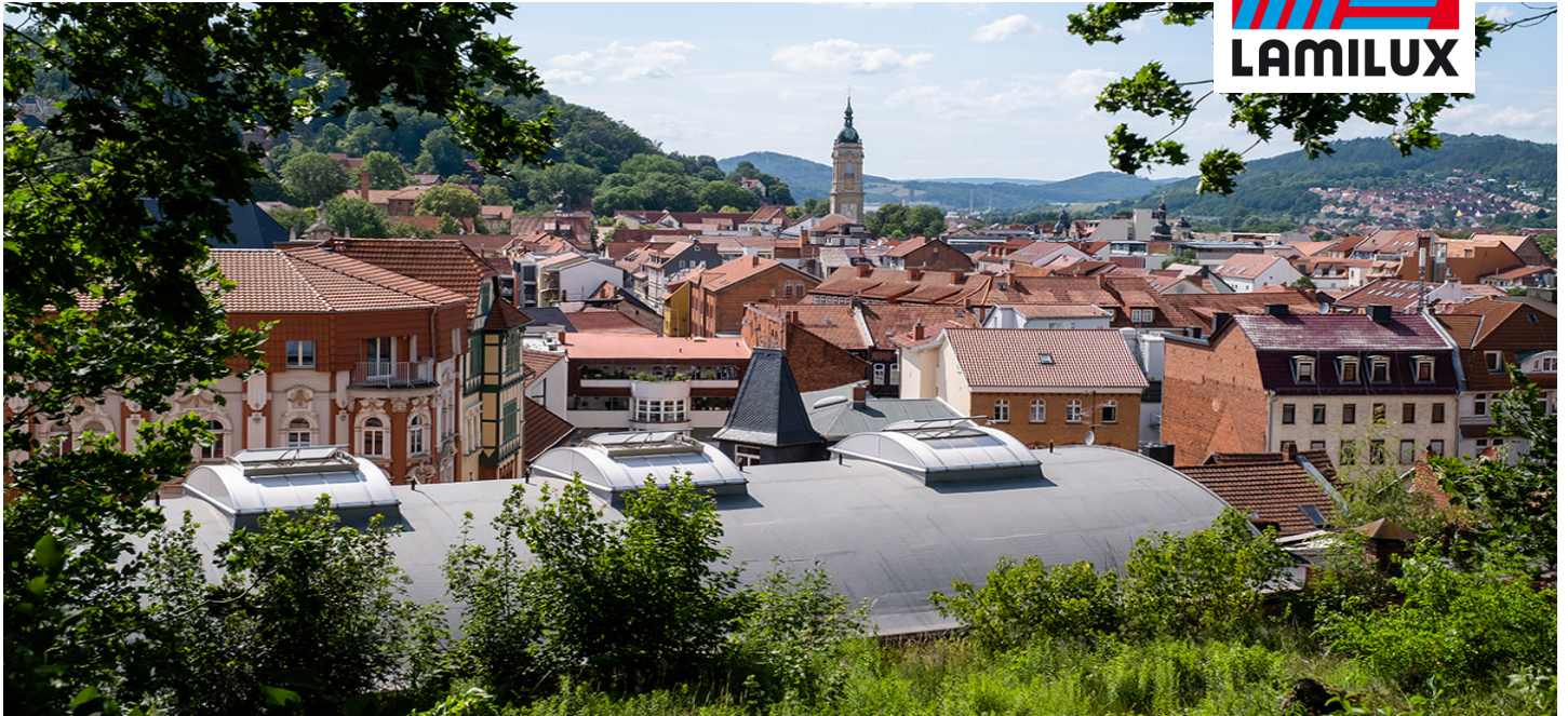
Climbing Hall, Eisenach (Germany)
